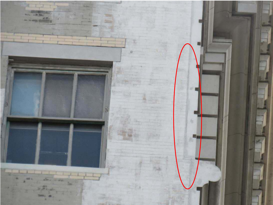
Photo: P079 Date 9/25/2017
