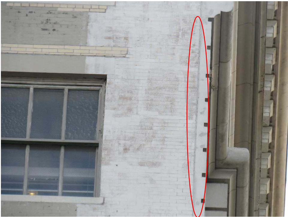
Photo: P080 Date 9/25/2017
