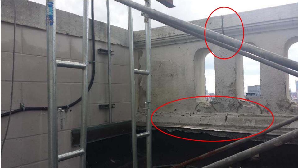
Photo: P100 Date 9/25/2017
