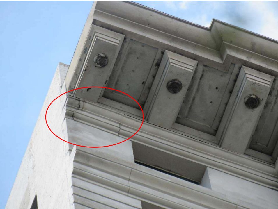
Photo: P001 Date 9/25/2017
