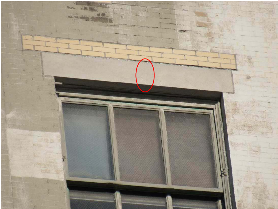
Photo: P082 Date 9/25/2017
