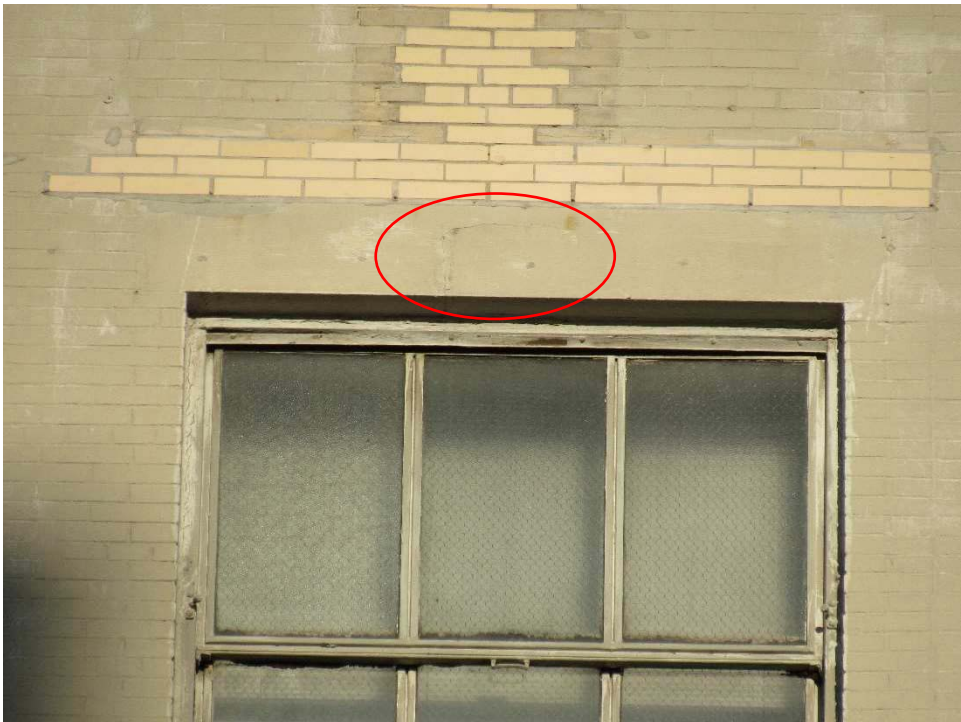
Photo: P046 Date 9/25/2017
