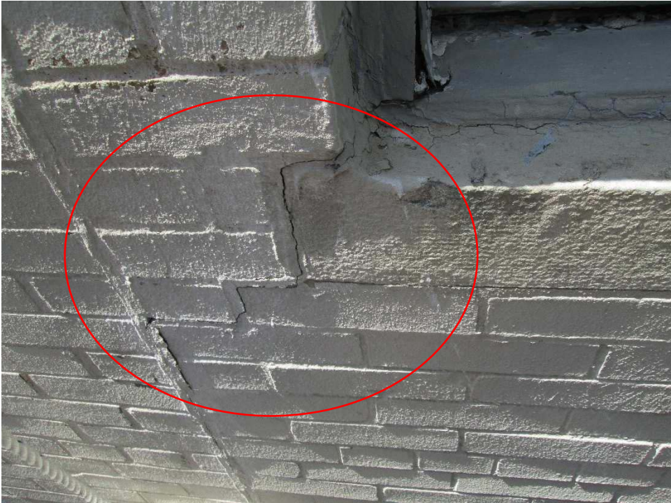
Photo: P036 Date 9/25/2017
