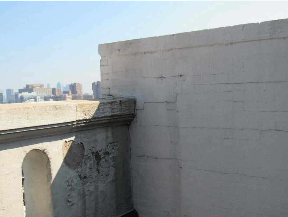
Photo: P099 Date 9/25/2017
