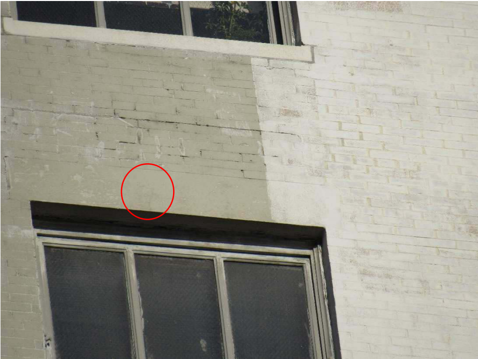
Photo: P081 Date 9/25/2017
