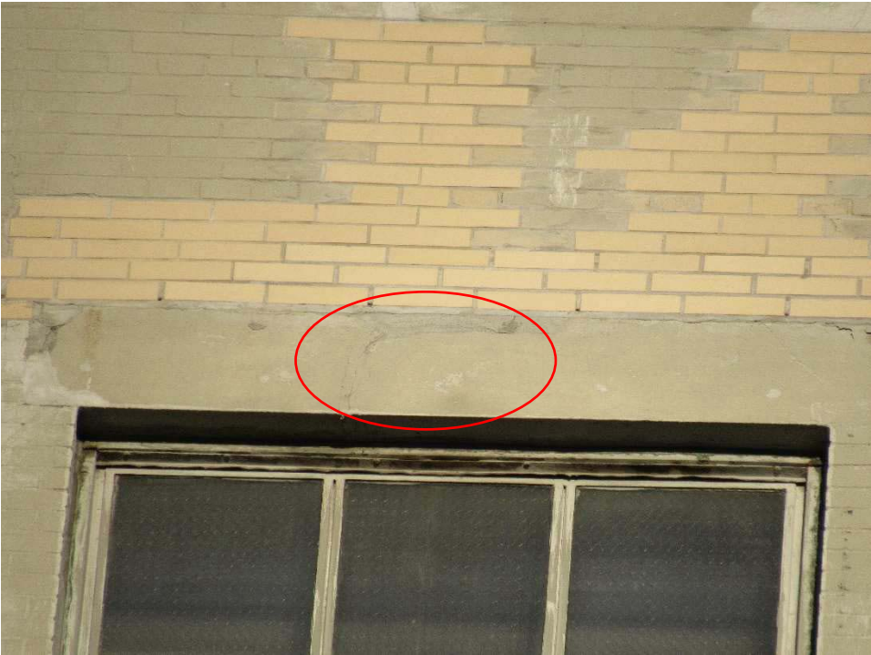
Photo: P045 Date 9/25/2017
