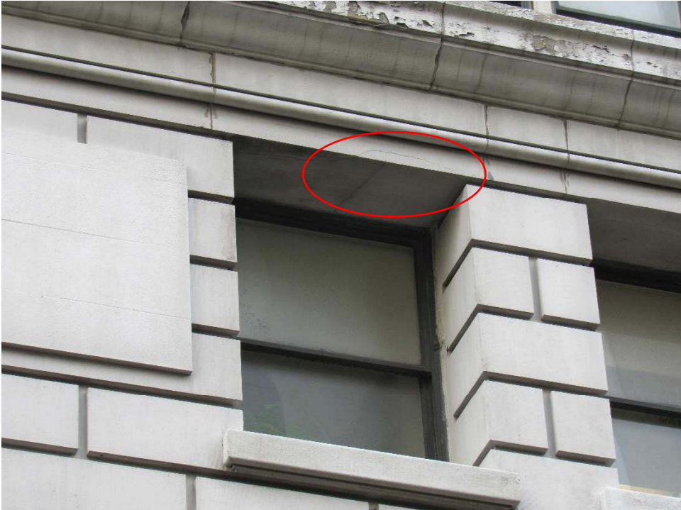
Photo: P002 Date 9/25/2017
