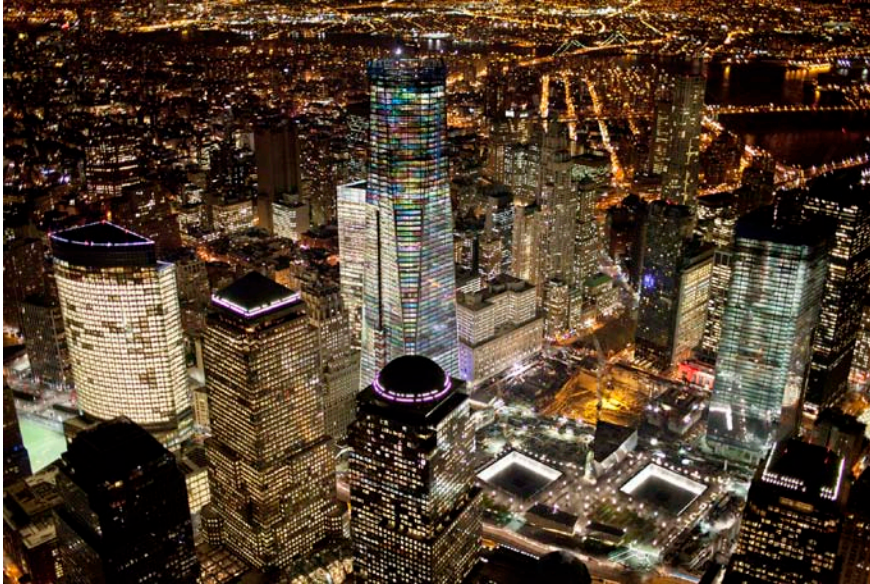
World Trade Center in Downtown Manhattan due to be completed in 2013.
