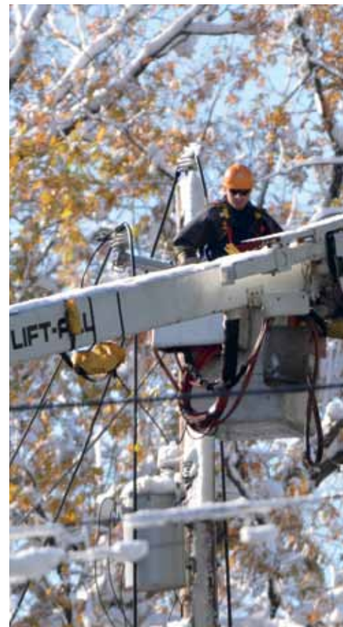
(Left) Operating Supervisor Heena Patel and Maintenance Supervisor Lauren Fox work on the steam system. (Top) Mechanic Karlos Diaz and Manager Gina Callender conduct substation job briefing. (Bottom) O&R Line Technician Jon Reiser restores service after October snowstorm.
