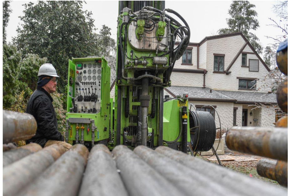
Geothermal heating system installation in Scarsdale NY
