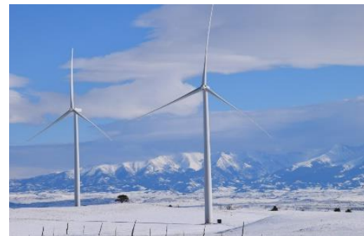
Big Timber Wind Project - Located in Montana
