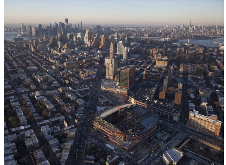
The Barclays Center sports and entertainment complex in Downtown Brooklyn is scheduled to be completed in September 2012.
