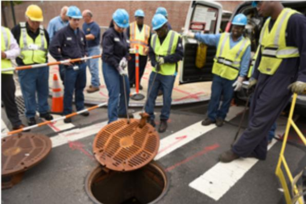
Con Edison workers test a latched manhole cover. The cover has a hinge on one side and latch on the other to allow heat and gases to escape without the cover dislodging.
