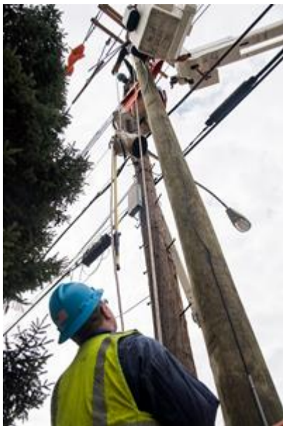
Con Edison crew members working on overhead lines in Westchester County.
