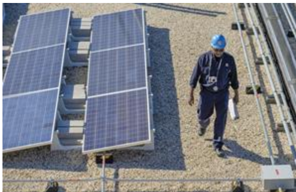
A Con Edison worker near solar panels atop a high school in Brooklyn.
