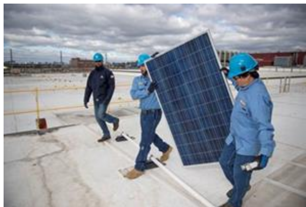
Con Edison workers carrying a solar panel on a company roof in Queens
